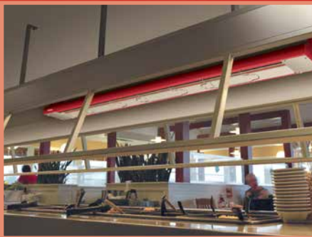
GRNH-48 with standard angle brackets and optional Designer color (sneeze guards shown not available) pg. 9
